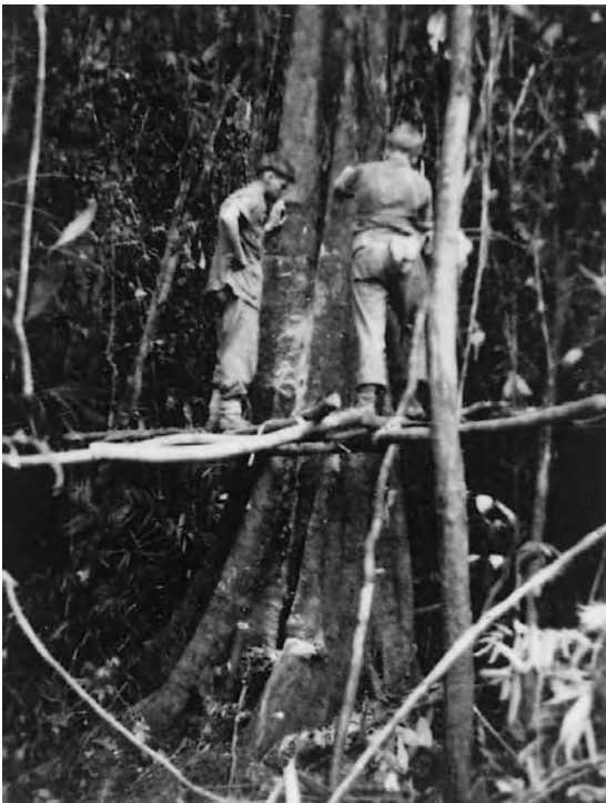
Tree felling for DZ. Sgt Hutton supervising, Rfn Mills sawing.
